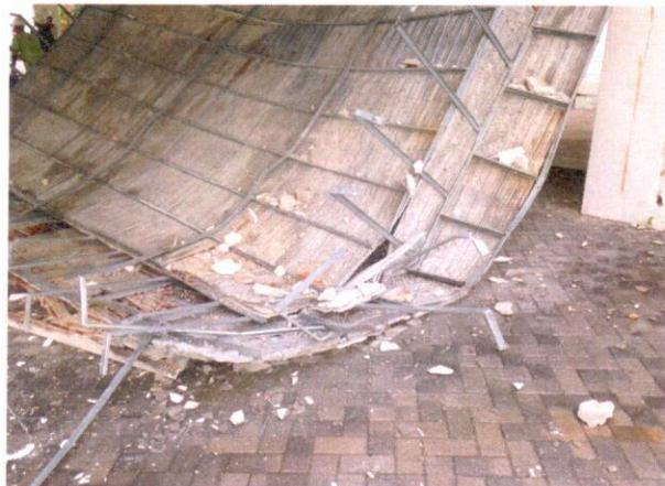
*Star Group has been removing the drop ceiling as directed by the engineer. They were working on the north side of this area and were ready to install shoring on this area. We could observe again that there were not enough supports holding the structure (see pictures).*
