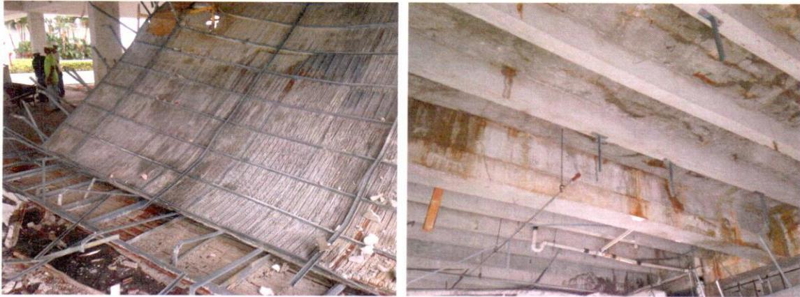
*We believe the lack of supports on the structure, the corrosion present on the supports due to several years of water leaks from the upper deck and the water increasing the weight of the stucco finish, have make the area collapse.*
